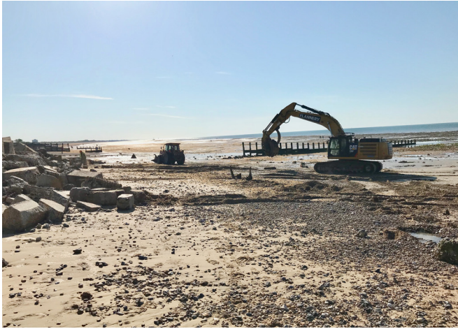
Environment Agency operatives completing public safety works in June
